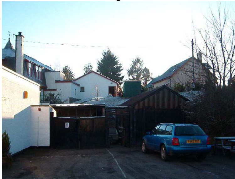
Fig 2 shows relationship between hotel extension to be demolished (centre) and new houses (right) to the west of the site.
